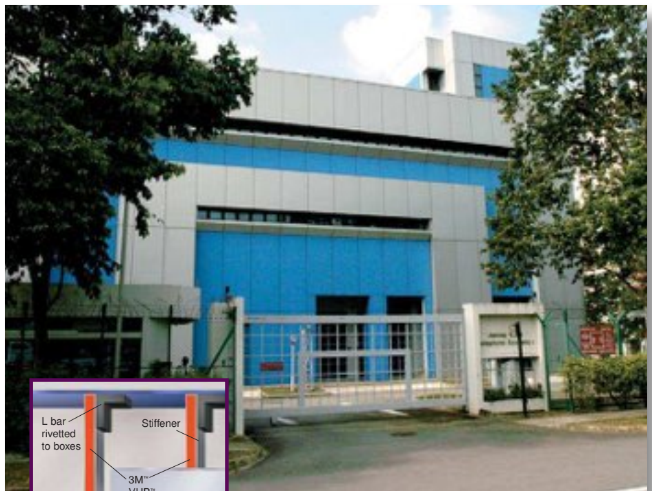
Jurong West Telephone Exchange, Singapore ACM panels attached to stiffeners.
