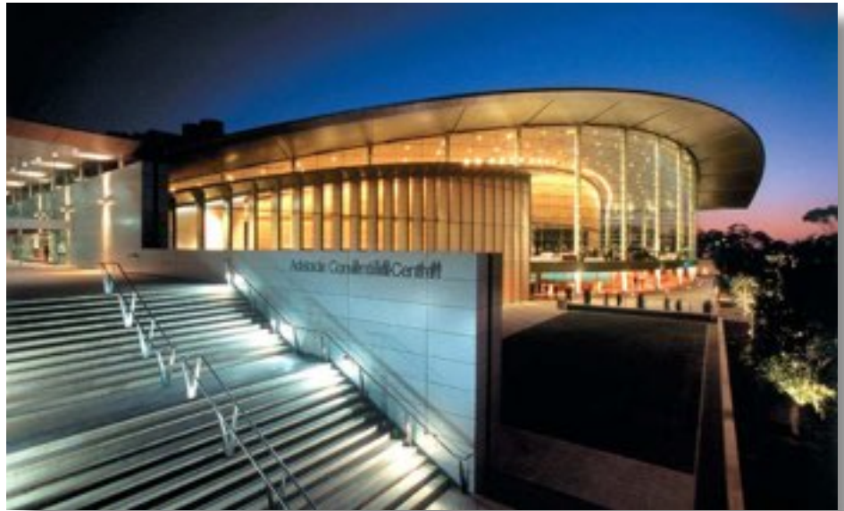
Adelaide Convention Centre, South Australia Architect: Woods Bagot with Skidmore, Owings & Merrill, 2001 Aluminum composite panel bonded to galvanized frame.
