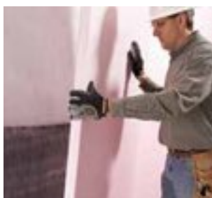
For fast, easy foam board installation, simply spray and stick with 3M™ Scotch-Weld™ Cylinder Spray Adhesive Holdfast 70. Bonds foam to concrete, waterproofing and more, without damaging the foam.
