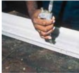
To prevent moisture penetration, a pressure flow gun applies 3M™ Scotch-Weld™ Nitrile High Performance Rubber and Gasket Adhesive 847 to a rubber gasket in a commercial light fixture cover.
