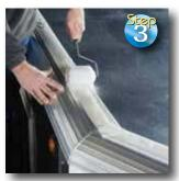
Roll down with a soft roller to conform over contours, seam edges, rivets or screw heads.
